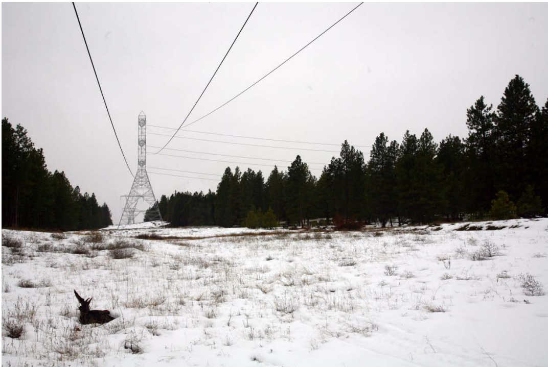
Figure 10b: Conceptual illustration from Viewpoint 10, where the proposed transmission line would tie into the existing BPA 345 kV transmission line from the intersection of its right-of-way and Loping Lane.
